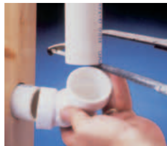
Damaged or leaking fitting is cut out
