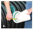
Measure the depth of the fitting to be attached to the pipe stub.
