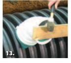
Install pipe fitting. Fitting should sit flush with the surface of the QwikSeal.
