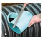
Bevel the leading edge of the pipe stub for easier insertion into the QwikSeal.
