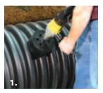
Core a perpendicular hole to the main line:
