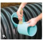
Lubricate the QwikSeal and pipe stub.
