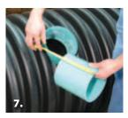
Add the dimensions of the QwikSeal and the fitting and cut a stub to that length.
