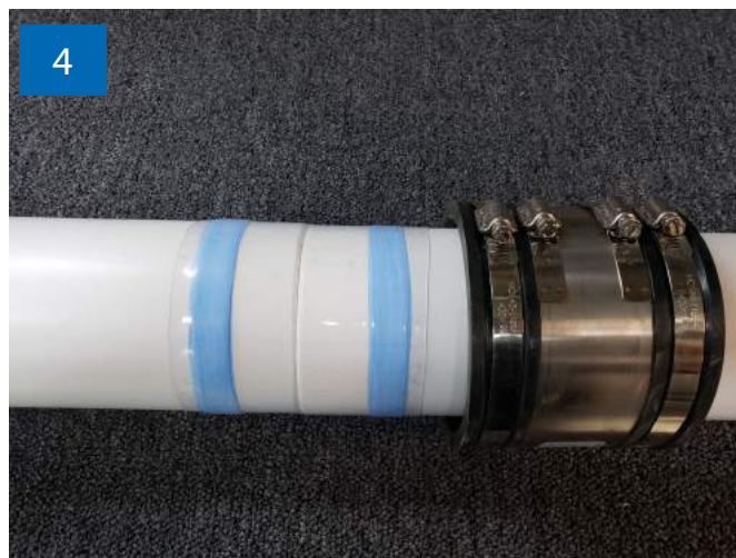
Center the FEP liner over the pipe ends and PTFE tape. Use heat gun to fully shrink the liner.
