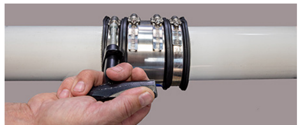
7. Ensure all bands are tightened to 60 inch pound.
