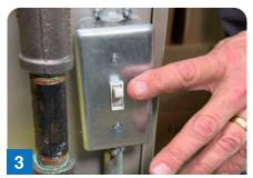
TURN POWER OFF Switch off power directly at the HVAC unit or the corresponding circuit breaker.
