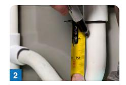
Measure 3/4" down from the dry fit mark and make a 2nd mark at each end. <u>This is where you will cut.</u>
