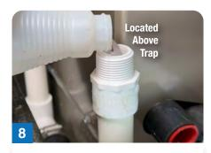
Prime the trap by pouring 3-6 ounces of tap water directly into the line.
