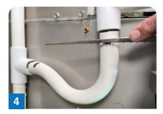
Using a PVC pipe cutter or hand saw, cut directly over the 2nd mark on each end and remove the old trap.
