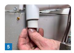
Using a utility knife or deburring tool, scrape away plastic fragments or burrs.
