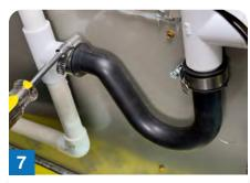
Slide each end of the new condensate trap over the corresponding pipe. Hand tighten with a nut or screw driver.
