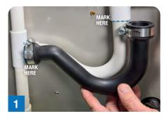
Dry fit the new condensate trap to ensure correct fit. Mark parallel lines on the existing pipe matching both ends of the new trap.
