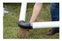
**Step 10** Add support blocks under each connection point to aid flow. Inspect for leaks.
