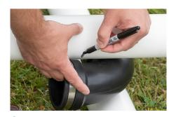
**Step 6** Measure both sections of the pipe using the end of the coupling socket as a guide.
