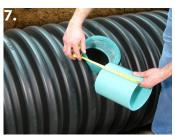
Add the dimensions of the QwikSeal and the fitting and cut a stub to that length.
