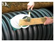
Install pipe fitting. Fitting should sit flush with the surface of the QwikSeal.
