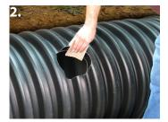
Using sand paper or a file, clean and remove any burrs from opening.
