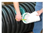
Measure the depth of the fitting to be attached pipe stub. See alternative method below.
