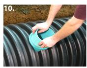
Start the pipe stub into the QwikSeal by hand.
