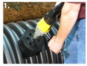
Core a perpendicular hole to the main line:
