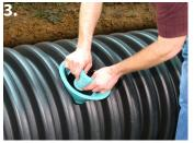
Remove band clamp from QwikSeal, fold and insert into opening. Unfold.
