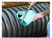
Bevel the leading edge of the pipe stub for easier insertion into the OwikSeal.
