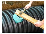
Using a hammer and block of wood, drive the pipe stub to the QwikSeal pipe stop.
