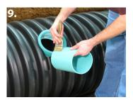
Lubricate the QwikSeal and pipe stub.
