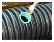
Measure the depth of the QwikSeal, from the pipe stop to the top edge.
