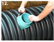
Install the band clamp at 60 in-lbs. torque.
