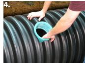
Pull up on QwikSeal until it stops against the inside of the pipe.
